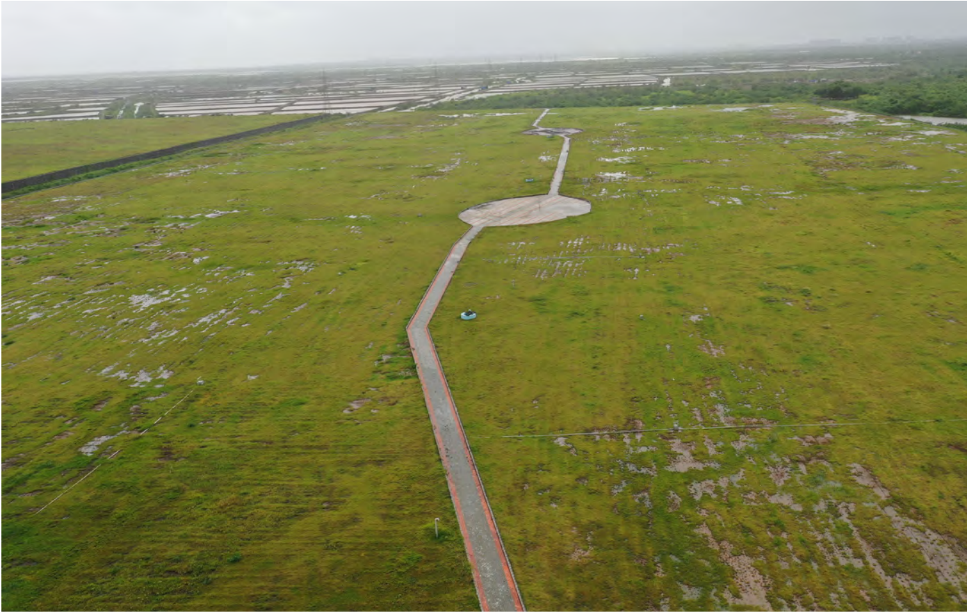
Bio-capped Khajod dumpsite
