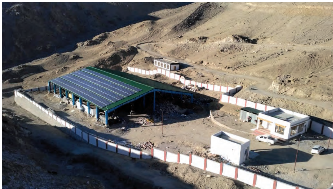
Solar panels installed on the roof of the plant supply sufficient energy for all mechanical operations
