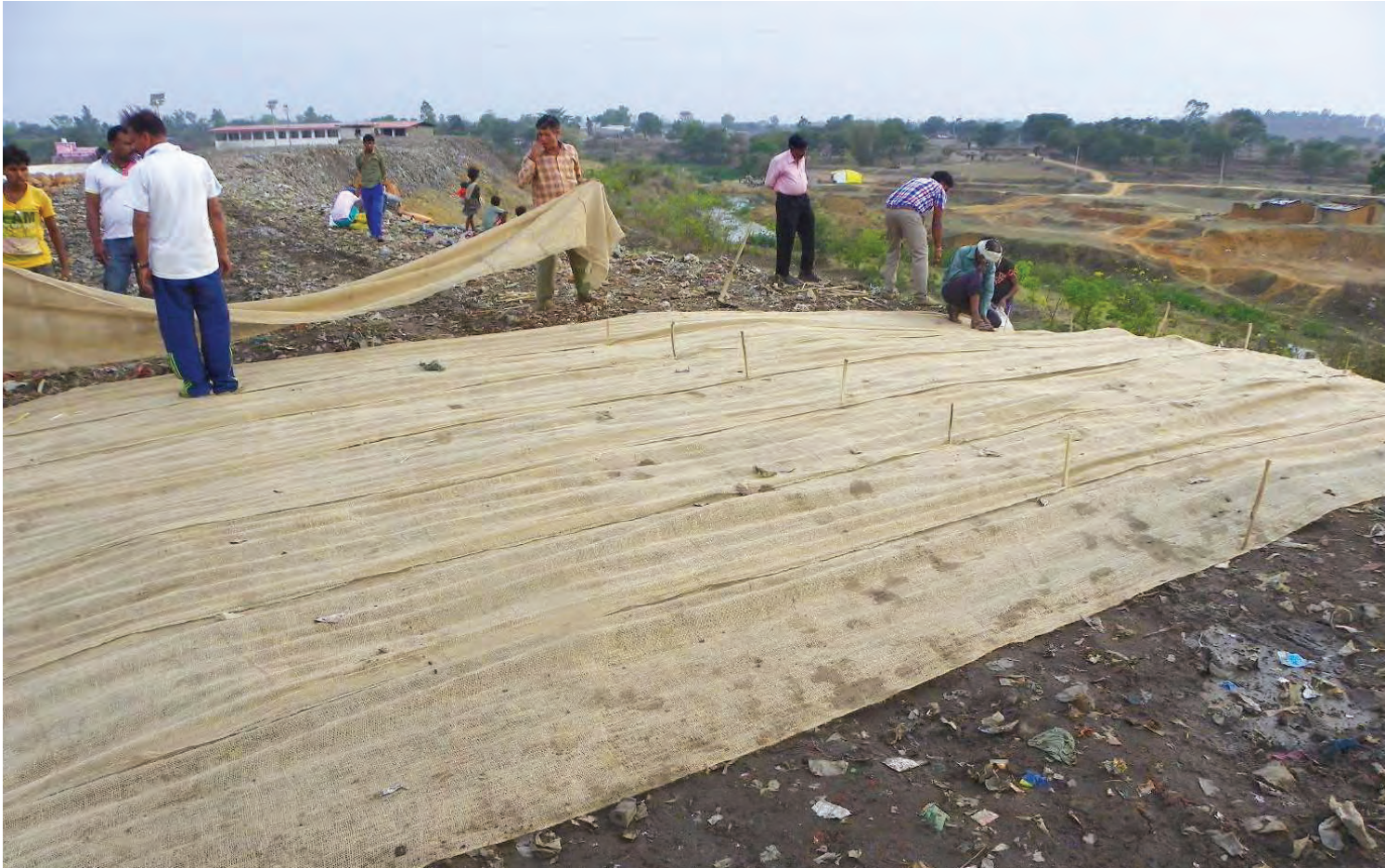
Legacy waste treatment: Jute capping, after which the entire waste surface is covered with capping materials like leaf mulch/organic manure/compost for two inches for cultivating local grass/ragi to bind the soil on the surface
