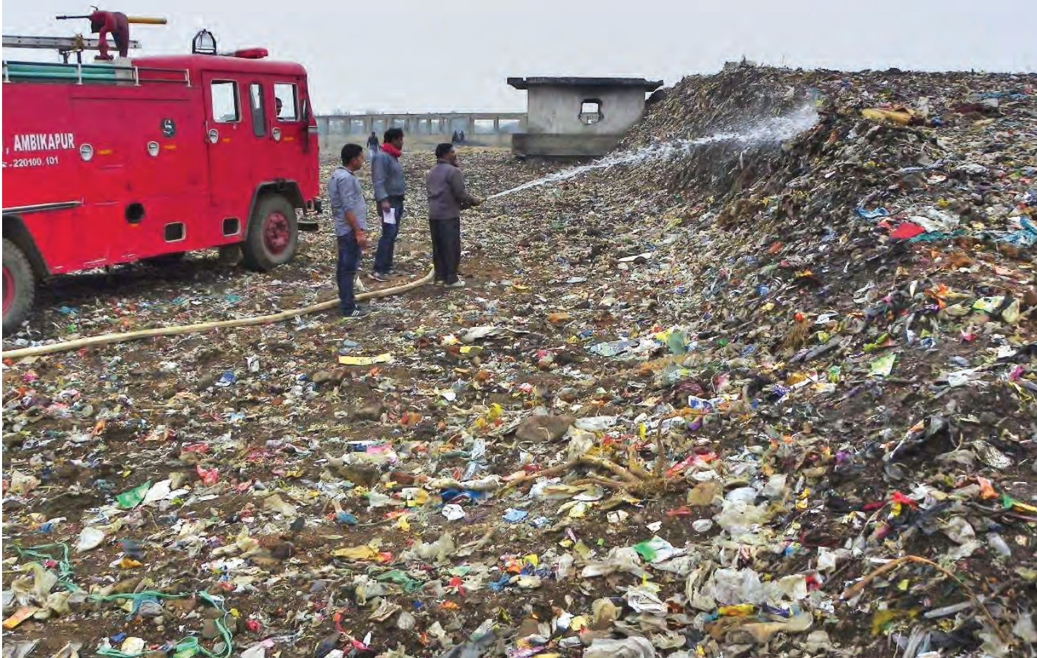
Legacy waste treatment: Sprinkling of water and bacterial inoculum – a minimum of 8 litre of water per tonne of mixed waste is required
