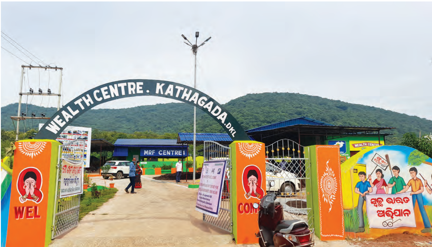
Waste processing facility at Kathagada
