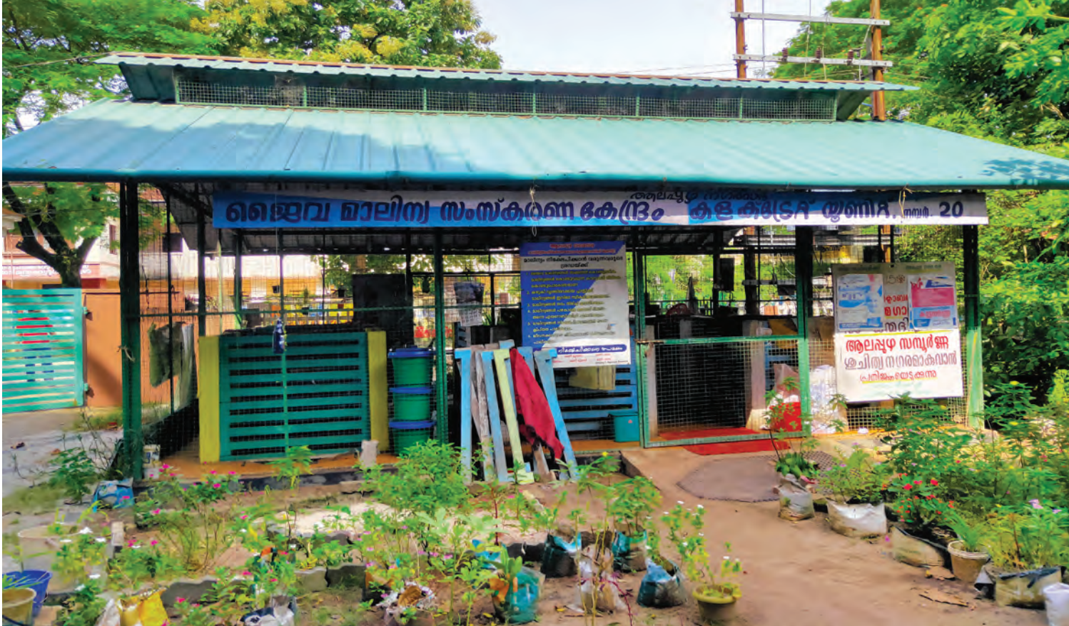
Biodegradable waste disposal center at Alappuzha district collectorate
