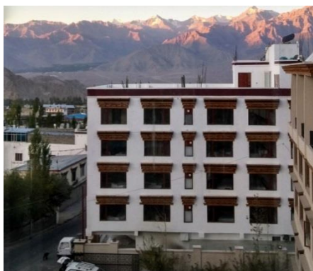
A modern building in Leh (Photo by Mani Juneja, TERI)
