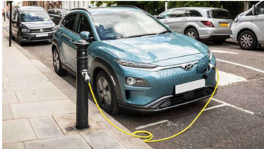
Figure 2.1: Hidden on-street charging points by Urban Foresight (GOV.UK, 2021)
